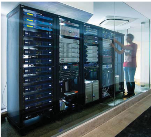
Central machine room
